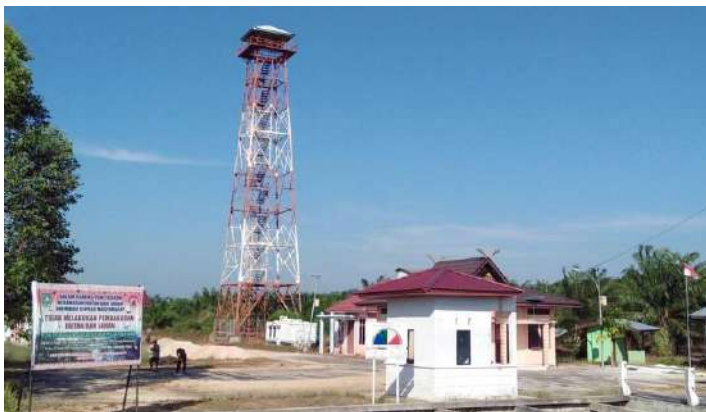
Figure 1. Integrated patrol post and fire monitoring tower in Desa Sepahat for coordination of fire prevention of MPA and stakeholders.
